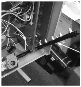
Rotate Valve/ Manifold Assembly
