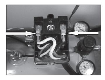
c. Take a 5/16" nut driver and remove the ground screws, holding down the ground wires.
