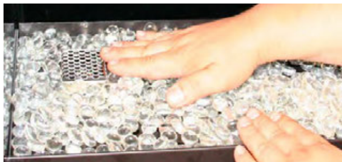
Figure 24a. Spreading the firestones evenly and make sure there are no firestones covering the pilot.
