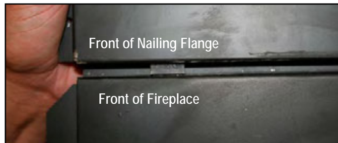
Figure 7b. Insert folded tabs into slots above the front of the fireplace
