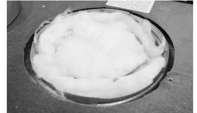
Step 3: Remove insulation from inside flue pipe.
