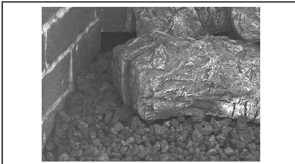
Figure 45: Installing the volcanic stone
