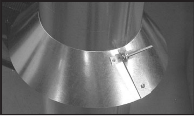
Figure 7.13 Insert Bolt into Brackets
