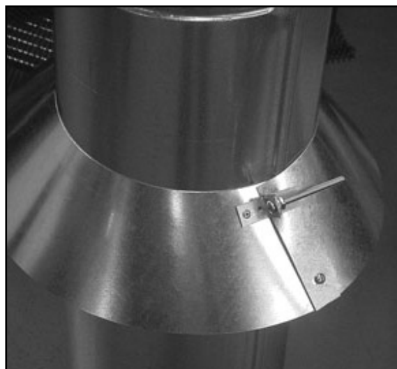
Figure 8.17 Assembling the Storm Collar Around the Pipe
