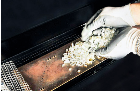
Spread the media evenly over the burner and media screens
