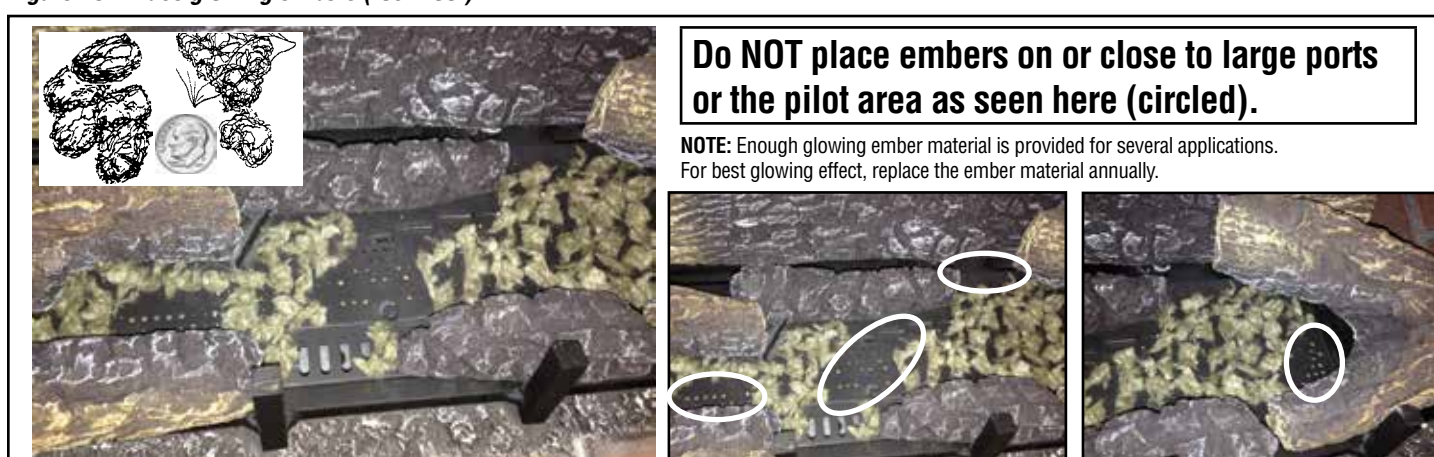
Figure 49 - Place glowing embers (rockwool)
