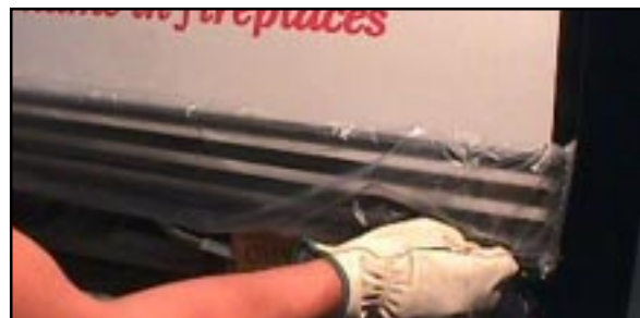
Figure 21 - Control Access Panel Removal
