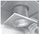
C. From inside the firebox, insert the 4" flue pipe / gasket assembly through the heat shield and out through the retaining ring. Secure the assembly to the rear and top of the appliance using 4 #8 x ¾" Hex Head Wildrill screws supplied. Do not overtighten. The gasket needs only to be snug against the firebox.
