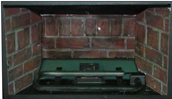
Figure 54: To remove the burner tube, gently pull it out of the venturi box.
