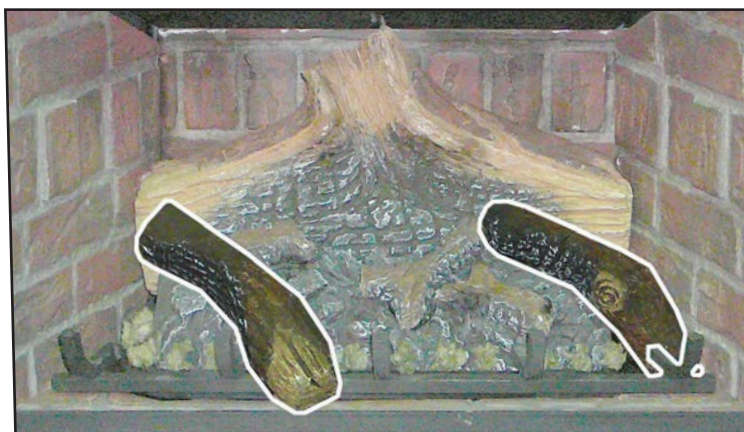
Figure 63: Fifth Stage Log Set Installation.
