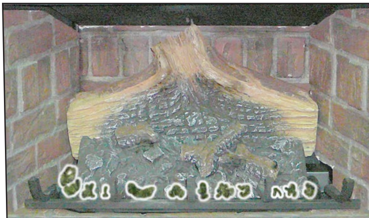
Figure 62: Fourth Stage Log Set Installation.
