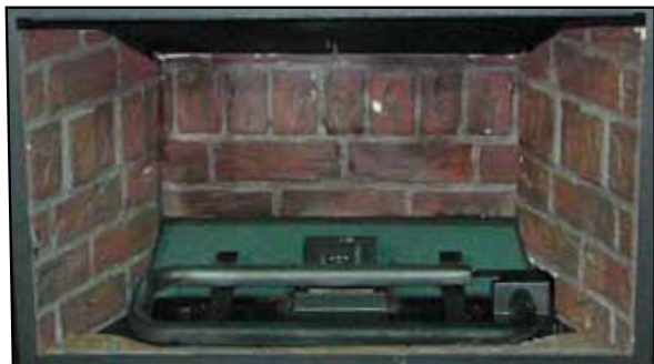
Figure 38: Carefully remove the front brick panel on the bottom of the firebox by lifting it up.
