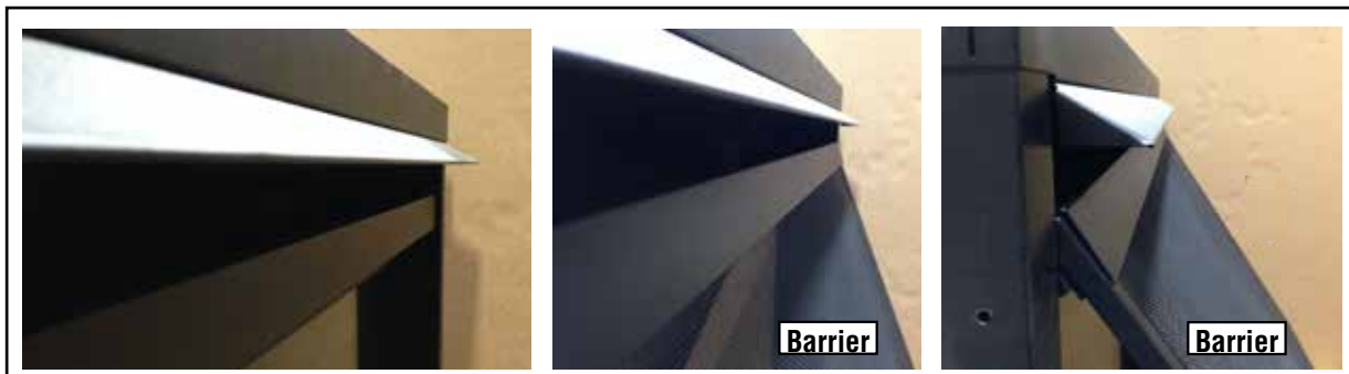
Figure 47A - Slide Barrier into Upper Trim Panel
