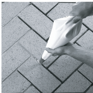
Figure 29 - Grouting Brick
