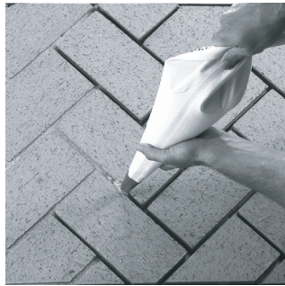
Figure 29 - Grouting Brick
