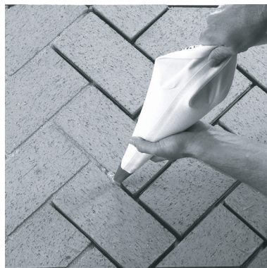
Figure 25 - Grouting Brick
